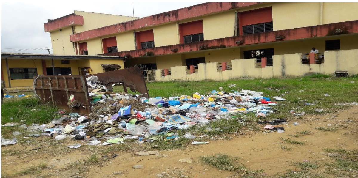
Plate 6: Broken waste receptacle inundated by plastic pollutants. Source: Researcher Field Survey 2021
